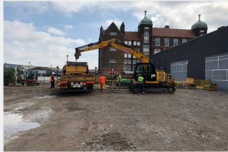
Piling Mat and Service Diversion Works Overview
